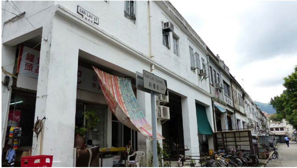
1. SKT-HB6-27 Front View (From No.22 to No. 1 San Lau St.)
